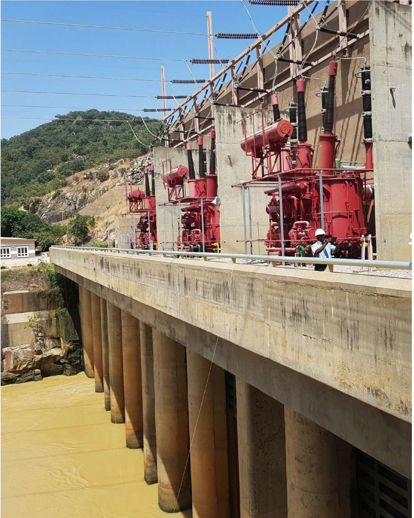
Shiroro Hydroelectric power station.
