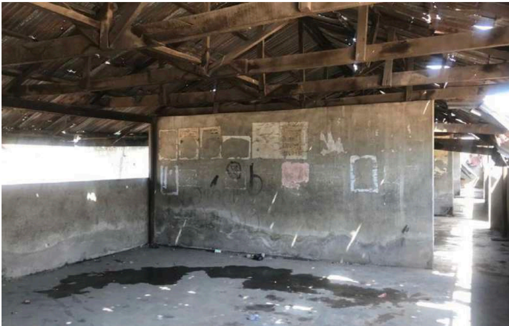
A section of the block of classroom before refurbishment by Stanbic IBTC
