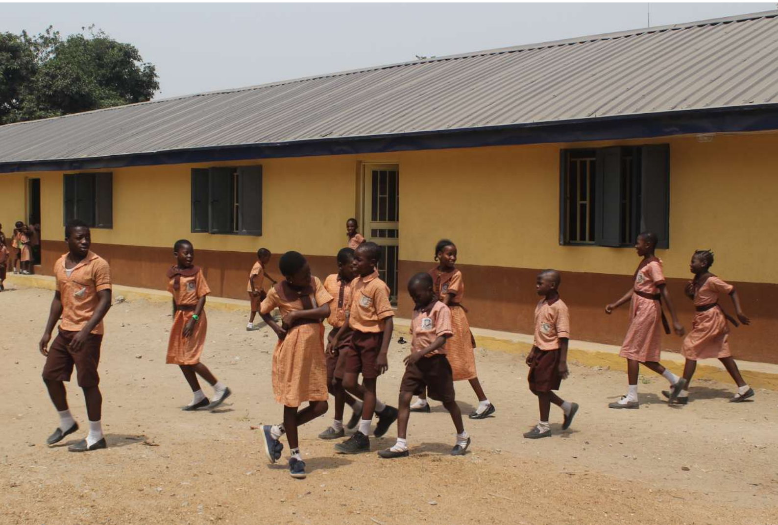
Refurbished block of classroom at Ladipo Primary School
